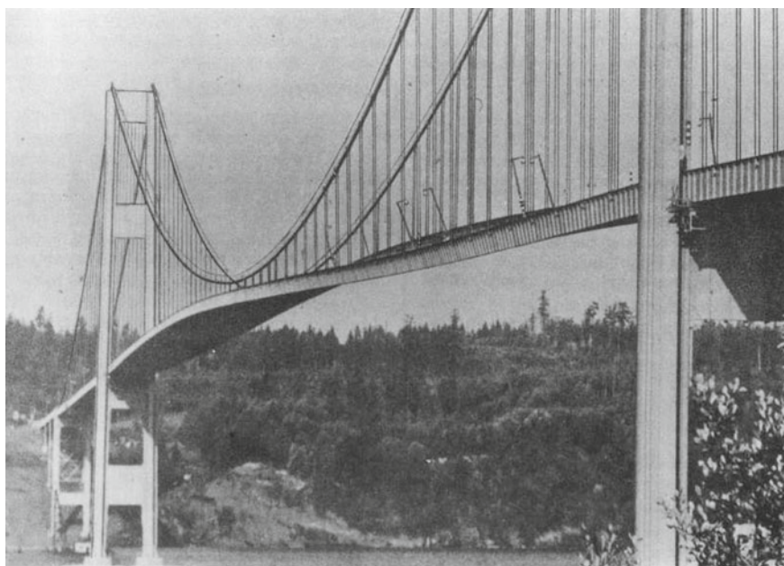
Fig. 6.2 Flutter of the Tacoma Narrows Bridge, November 10, 1940. From Farquharson FB (ed) Aerodynamic Stability of Suspension Bridges , 1949–1954
